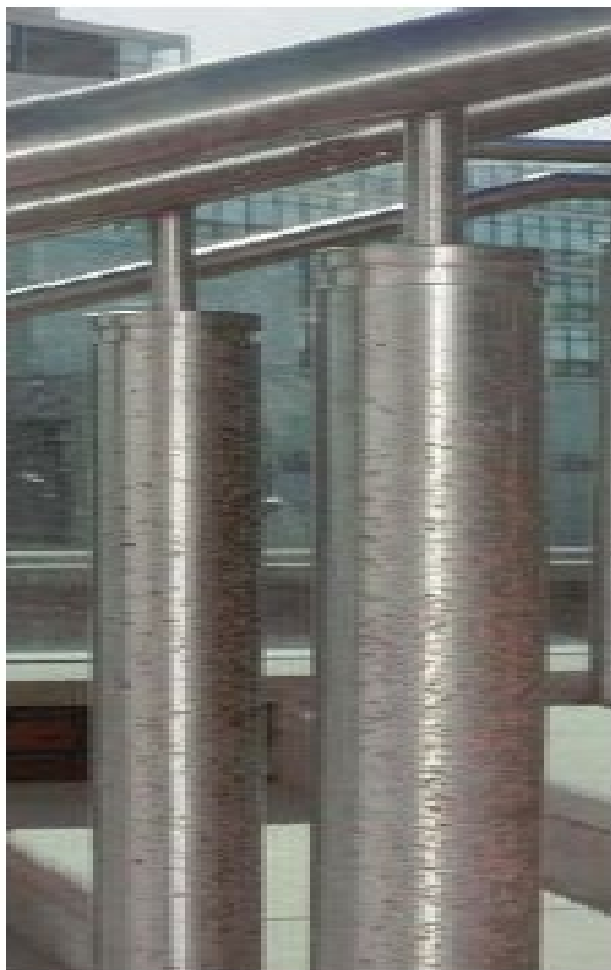
Rusting of iron contamination during the service life of stainless steel is unsightly. Removal can be time-consuming and expensive.
